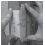
2b Peel adhesive backing and paste the folded template square to the frame
