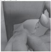
2c Cut the frame inside the unshaded area marked on the template. Install strike per installation instructions 24201428
