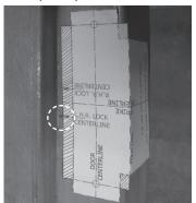
3c Cut the frame inside the unshaded area marked on the template. Follow mounting tab installation instructions. Install strike per installation instructions 24201428
